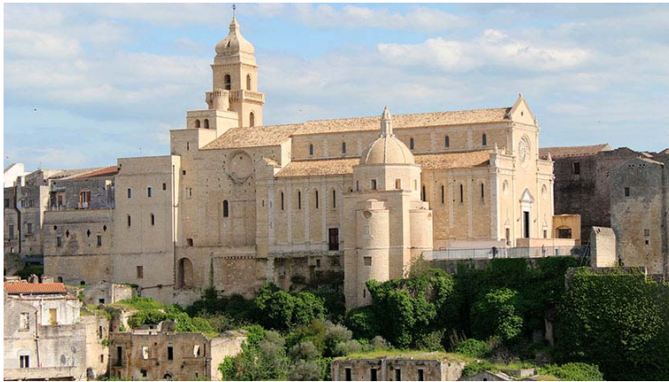
Fig. 1 S. Maria Assunta Cathedral, Historic center view of Gravina in Puglia
